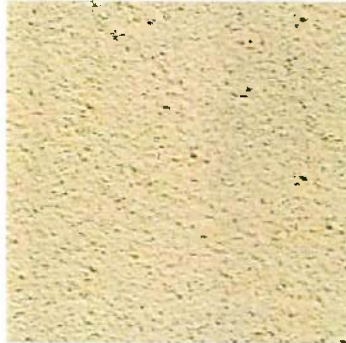
2 EXTERIOR CEMENT PLASTER LA HABRA - SAND FLIGHT 2020
